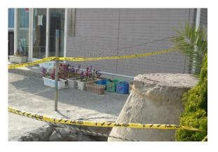
appeared in the ground, water pipes broke, and a manhole in front of the building popped up from the ground (please see the picture above).
